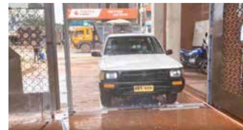
Automated car/vehicle disinfection system
